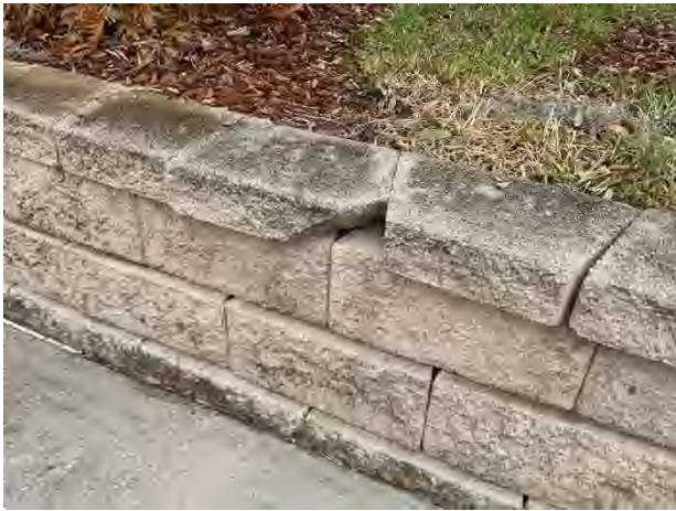
Masonry spall
