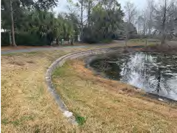
Masonry retaining wall
