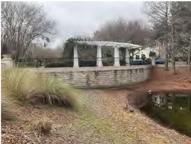
Masonry retaining wall
