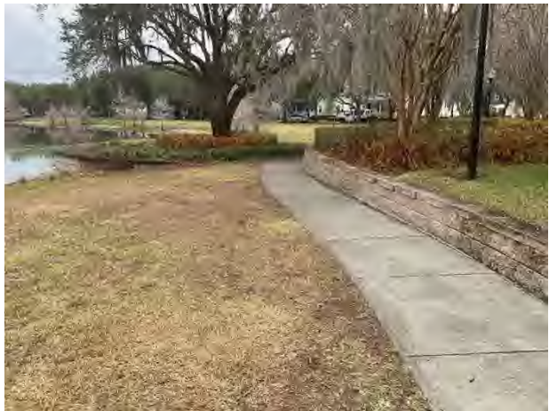
Masonry retaining wall
