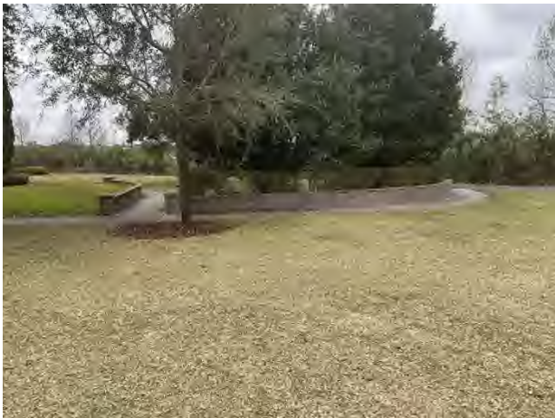
Masonry retaining wall
