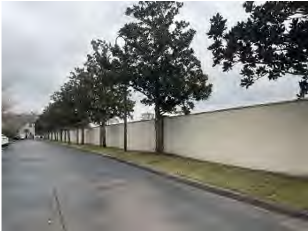
Concrete perimeter wall overview
