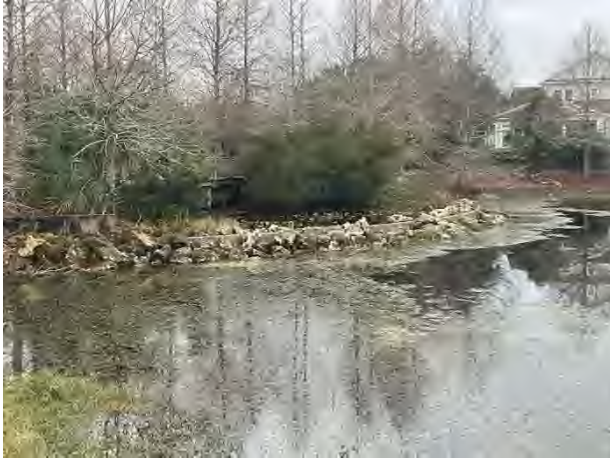
Rip rap and concrete weir
