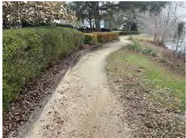
Masonry retaining wall
