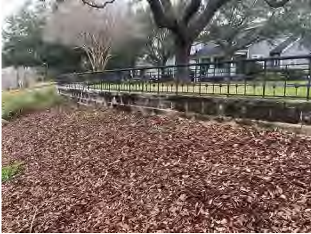
Masonry retaining wall
