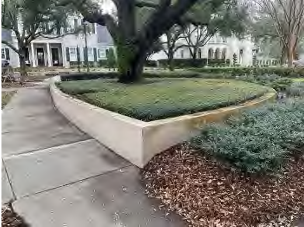
Concrete retaining wall
