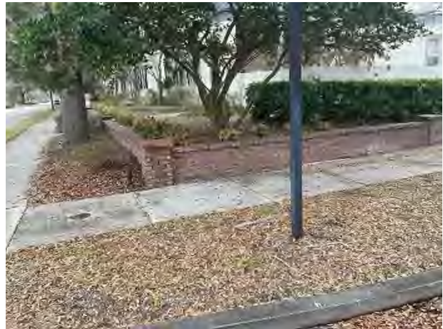
Masonry retaining wall
