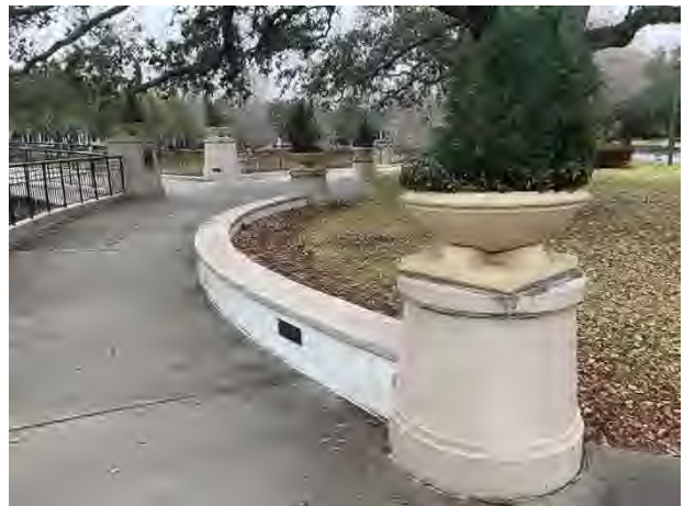
Concrete, retaining walls and planters
