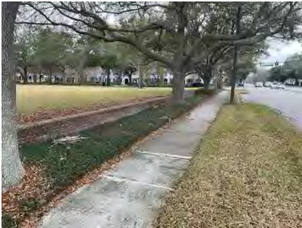
Masonry retaining wall
