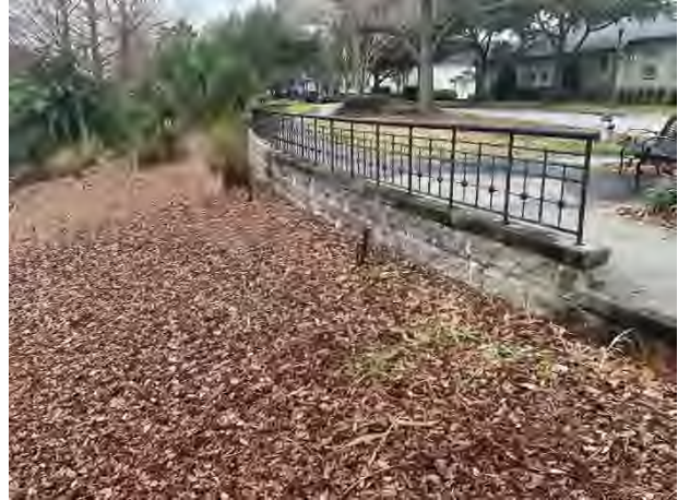
Masonry retaining wall
