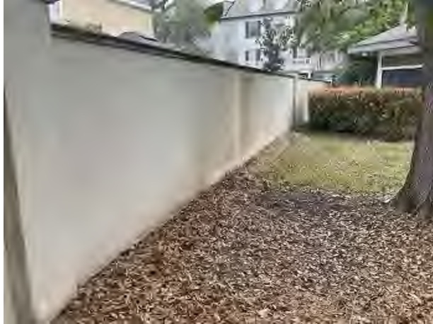
Finish deterioration
