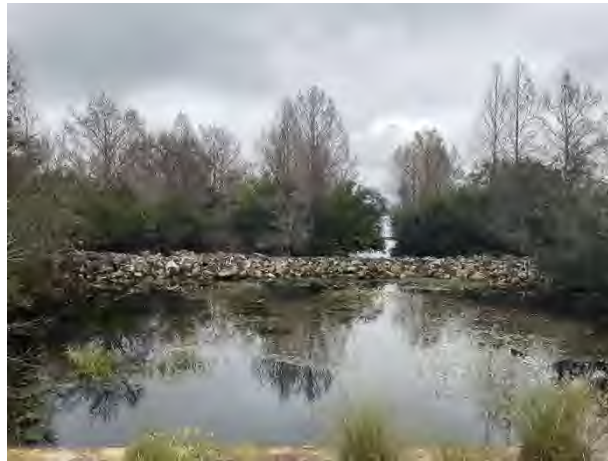
Rip rap and concrete weir
