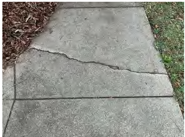
Sidewalk cracks
