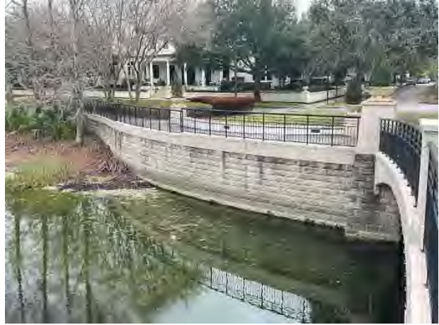
Masonry retaining wall
