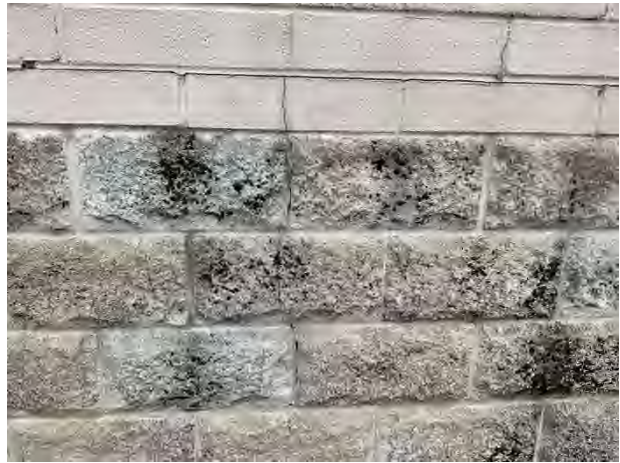
Masonry cracks
