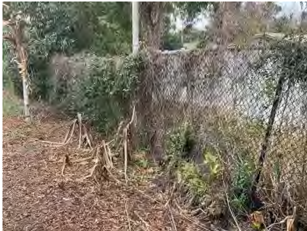
Chain link fence
