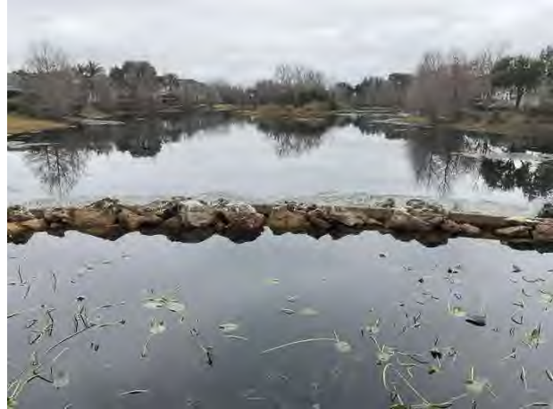
Rip rap and concrete weir
