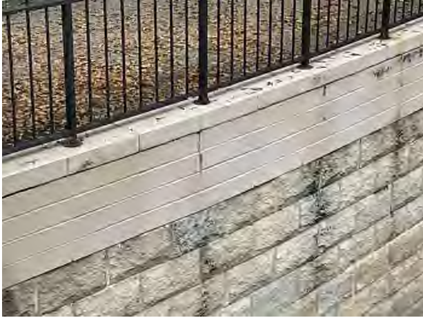
Masonry cracks
