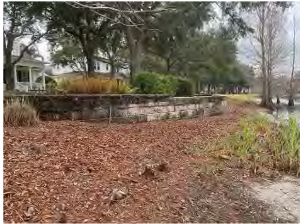
Masonry retaining wall
