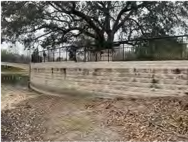
Masonry retaining wall
