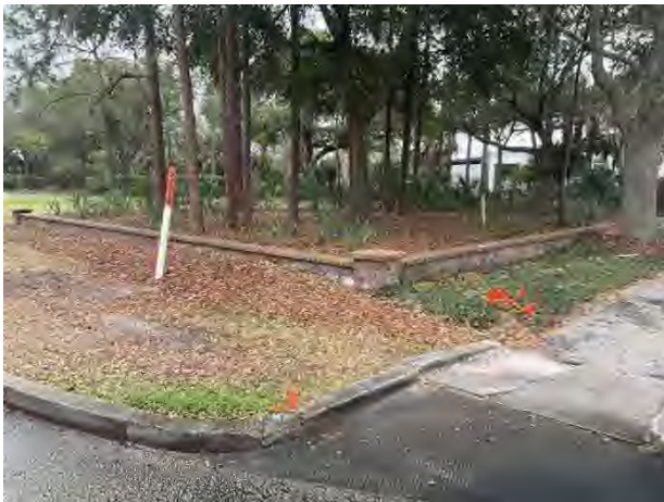
Masonry retaining wall
