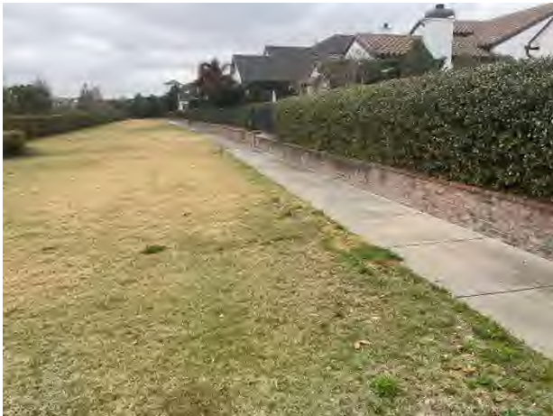
Masonry retaining wall
