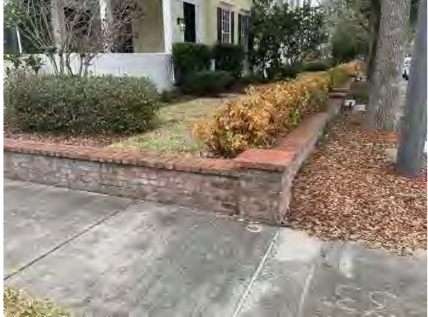
Masonry retaining wall
